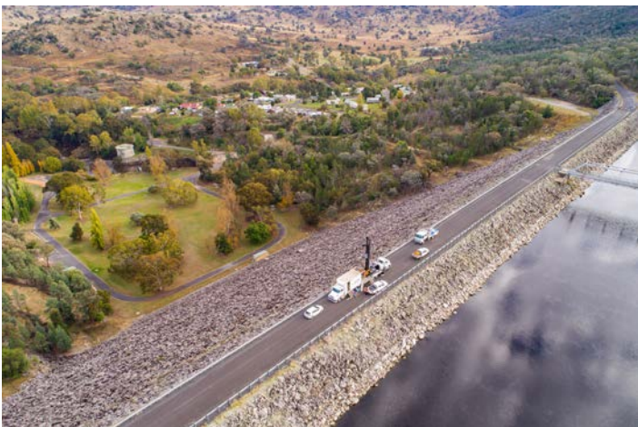
Geotechnical drilling at Wyangala Dam allows the project team to best inform design and planning. (The dam's road is closed during this testing).
