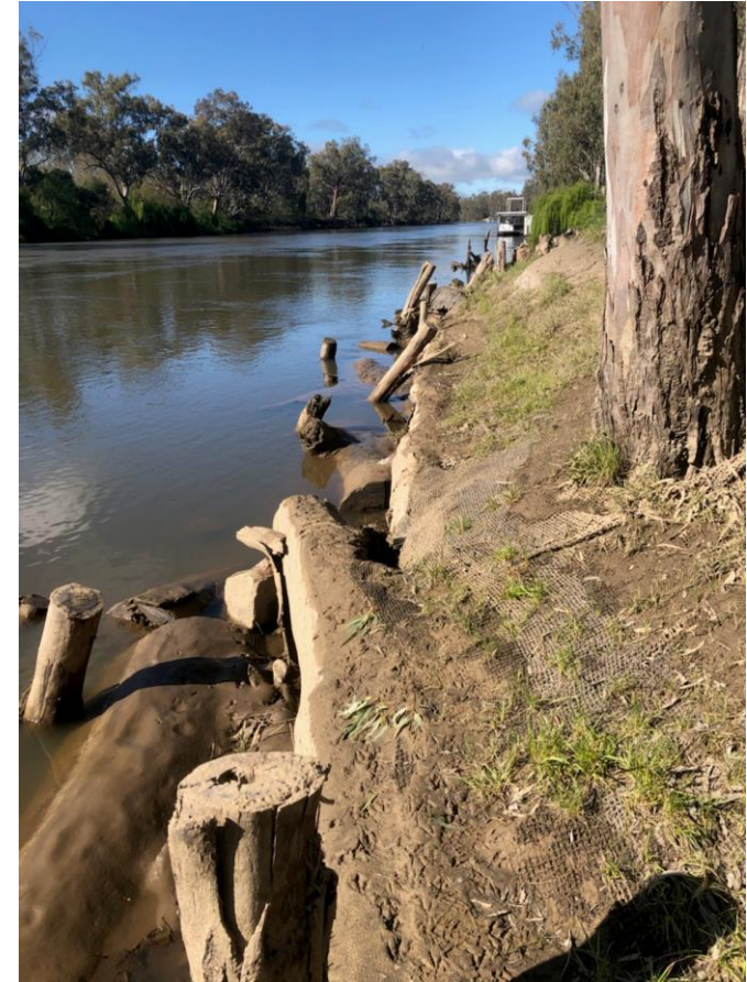
Murray River near Corowa - Deposition of sediment on log revetment sites following ~40,000 ML/d flow in Sep 2021 Photo: Ben Berry, Soil Conservation Service
