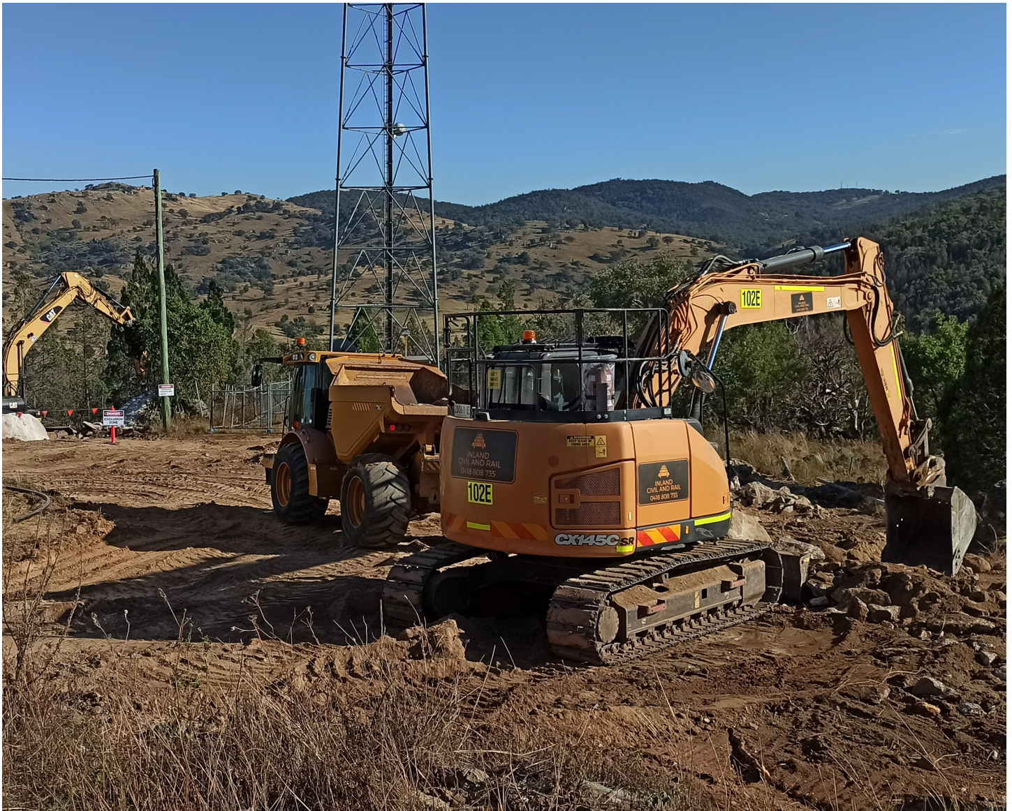
Clearing and leveling works, undertaken by RECS Group based in Young
