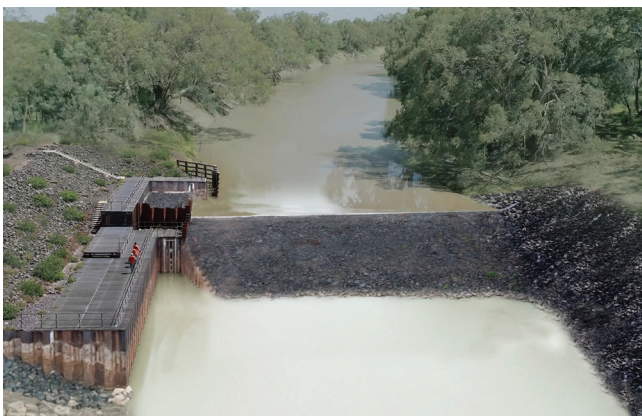
Artist impression of the new weir and fishway in normal flow mode.
