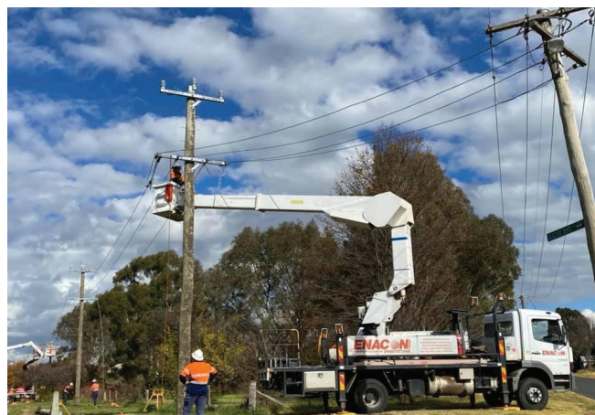
Enacon Group undertaking overhead electrical works on another project
