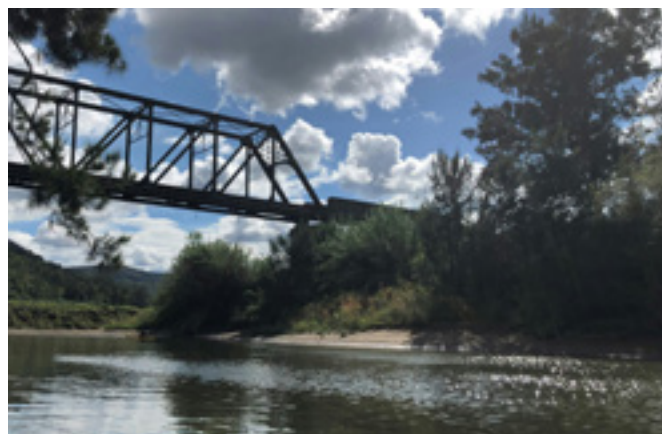
The Paterson River at the Paterson rail bridge looking upstream.
