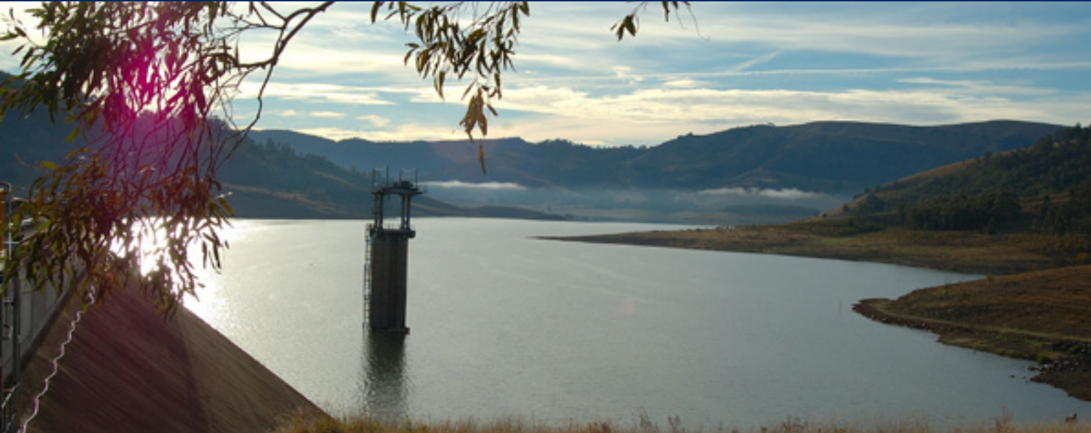
Glennies Creek Dam and surrounds. Image courtesy of WaterNSW.
