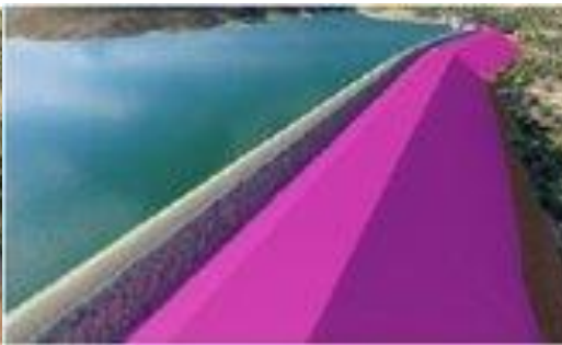
Stage 2 – Placing downstream rock fill
