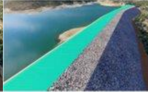
Stage 4 – Start raising dam wall
