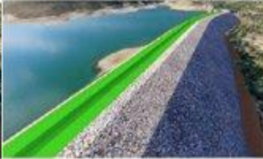
Stage 3 – Removing existing dam crest
