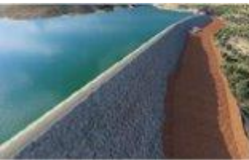
Stage 1 – Preparing downstream foundation
