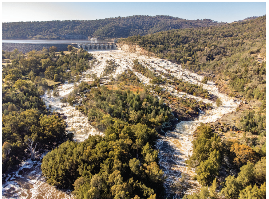
Wyangala Dam, photo by Farpix
